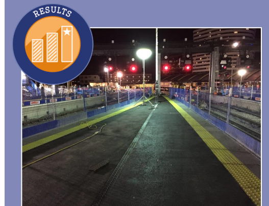
Resurfaced platform at Waterloo
